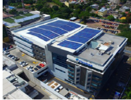
Plaza Victoria Building, Tegucigalpa
